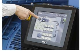
The new APM802 command/control system is specifically designed for operating and monitoring power plants for markets including hospitals, data centres, banks, the oil and gas sector, industries, IPP, rental and mining.
